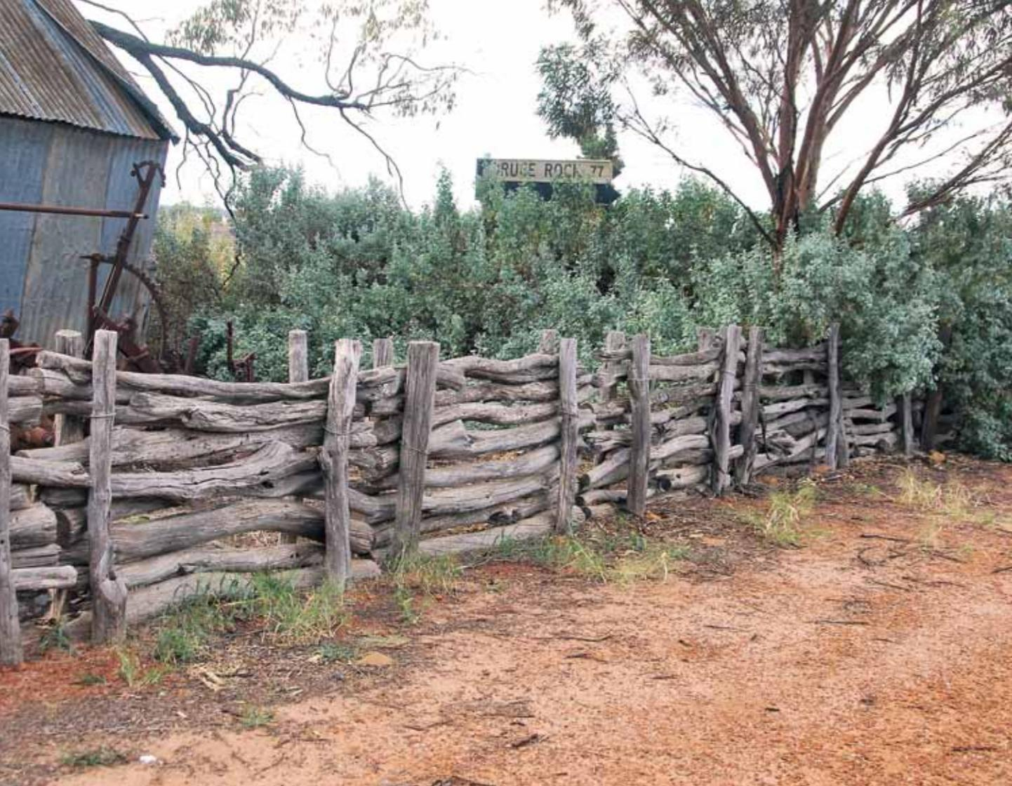
*This reconstructed fence at the old bakery, Greenhills, WA, is a variation of the Harper fence, constructed of separate panels rather than overlapping rails.*
