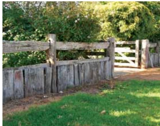
*A three-rail jarrah split rail fence near Pemberton, WA (left), and a hybrid split rail/paling fence at Perup, WA (right).*
